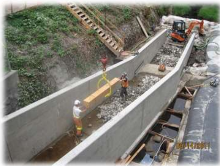
Metro Vancouver Cariboo Dam Fishway under Construction
