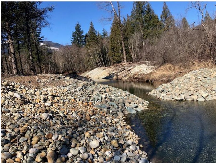
Photo 8 Looking north at William Phillips Slough Weir 2B (March 16, 2020).
