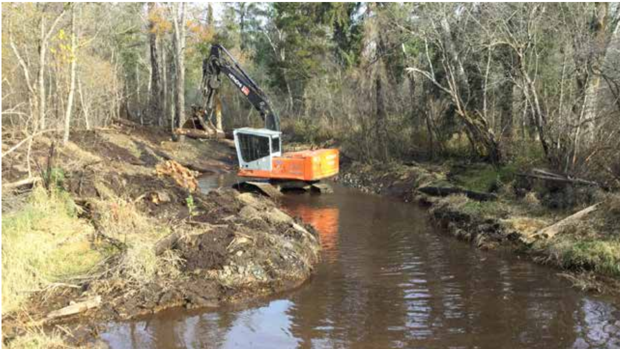
Photo 12 November 7, 2019 - Marhag construction placing LWD in Nancy Phillips Slough.
