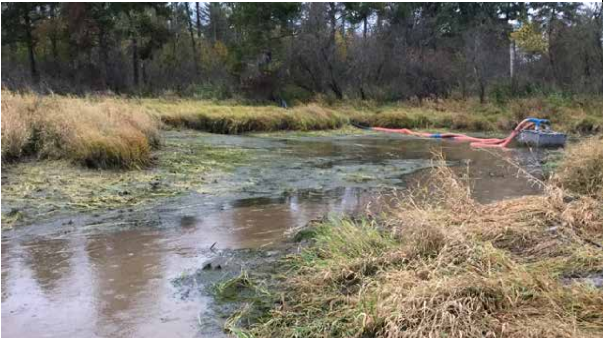
Photo 4 October 18, 2019 – Dewatering of work area at William Phillips Slough.
