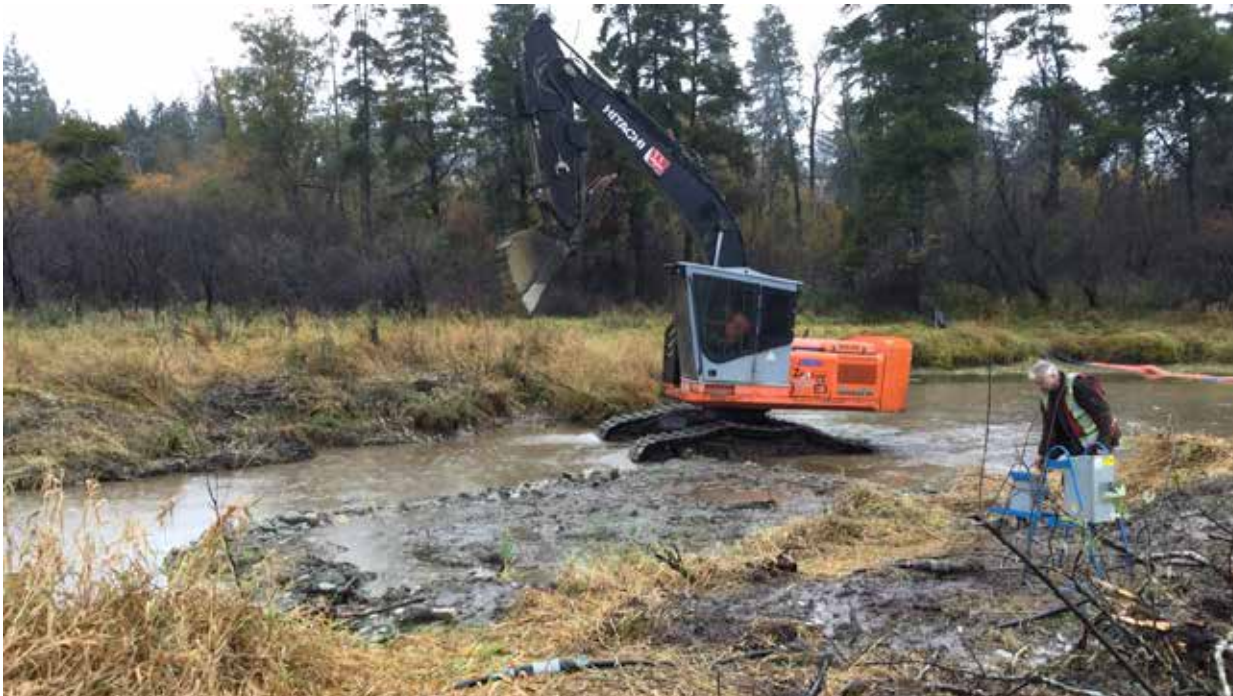
Photo 6 October 21, 2019 – Channel excavation at William Phillips Slough.
