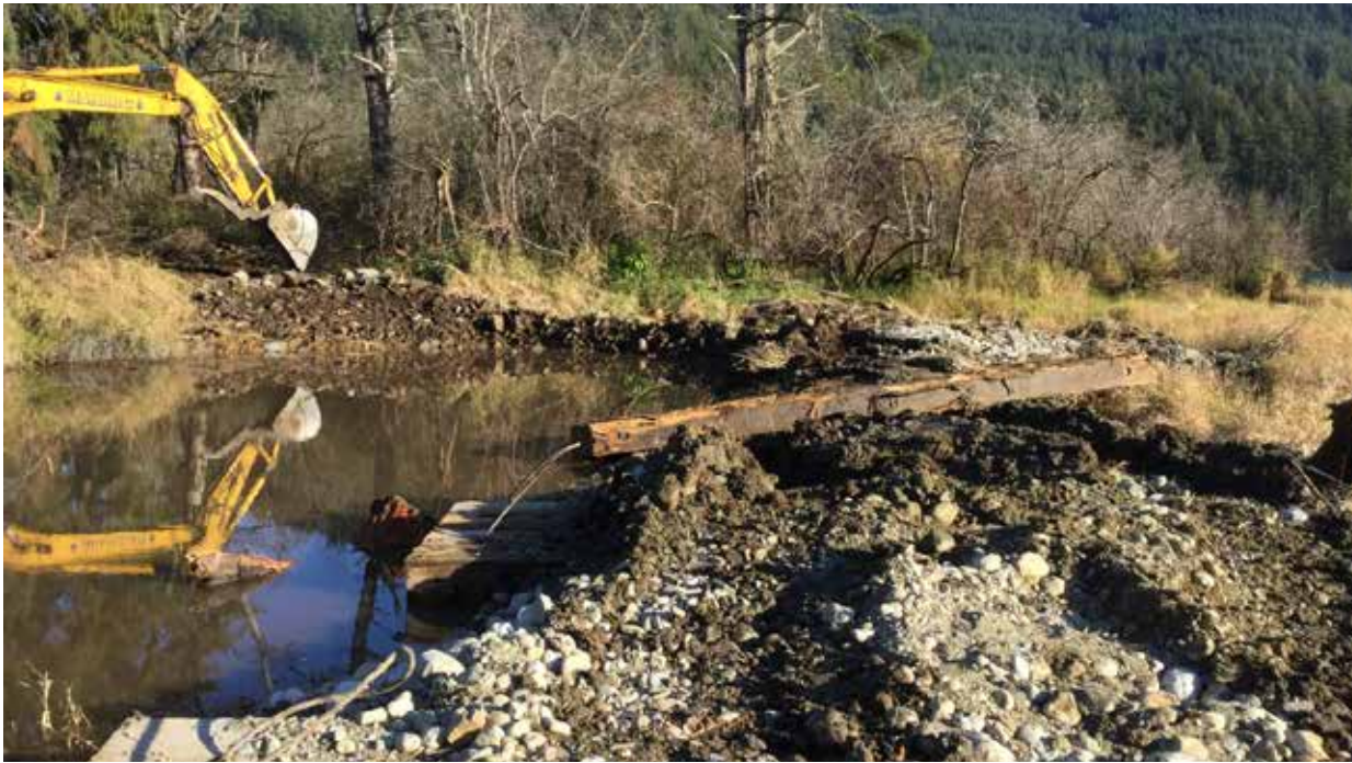
Photo 9 October 28, 2019 – LWD installed at William Phillips Slough
