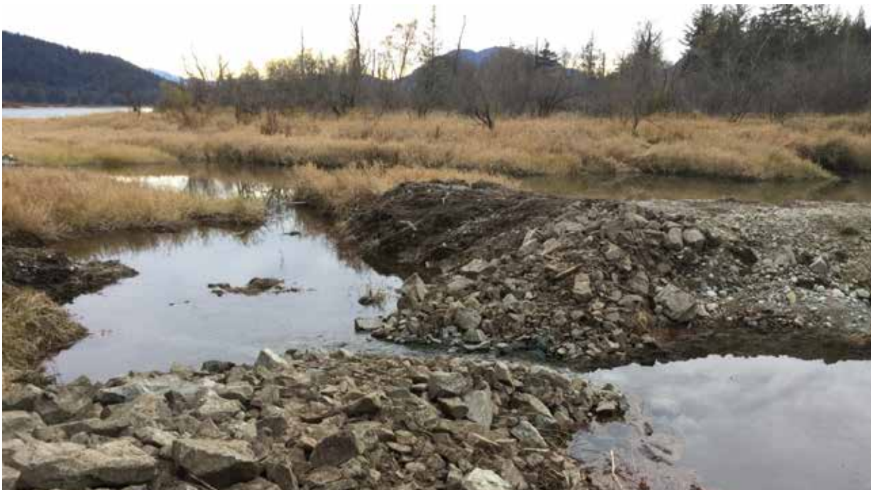
Photo 10 November 7, 2019 – West view of the downstream rock weir at William Phillips Slough.
