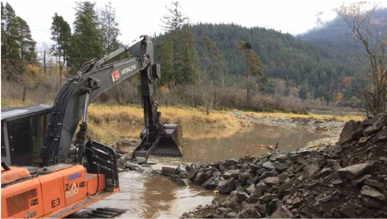
Photo 7 October 24, 2019 - Marhag equipment installing a rock weir on William Phillips Slough.
