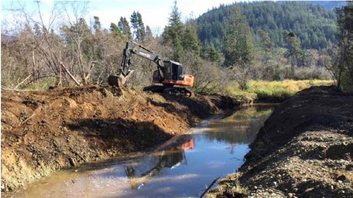
Photo 1 October 11, 2019 – Beginning of excavation of channel at Williams Phillips Slough.
