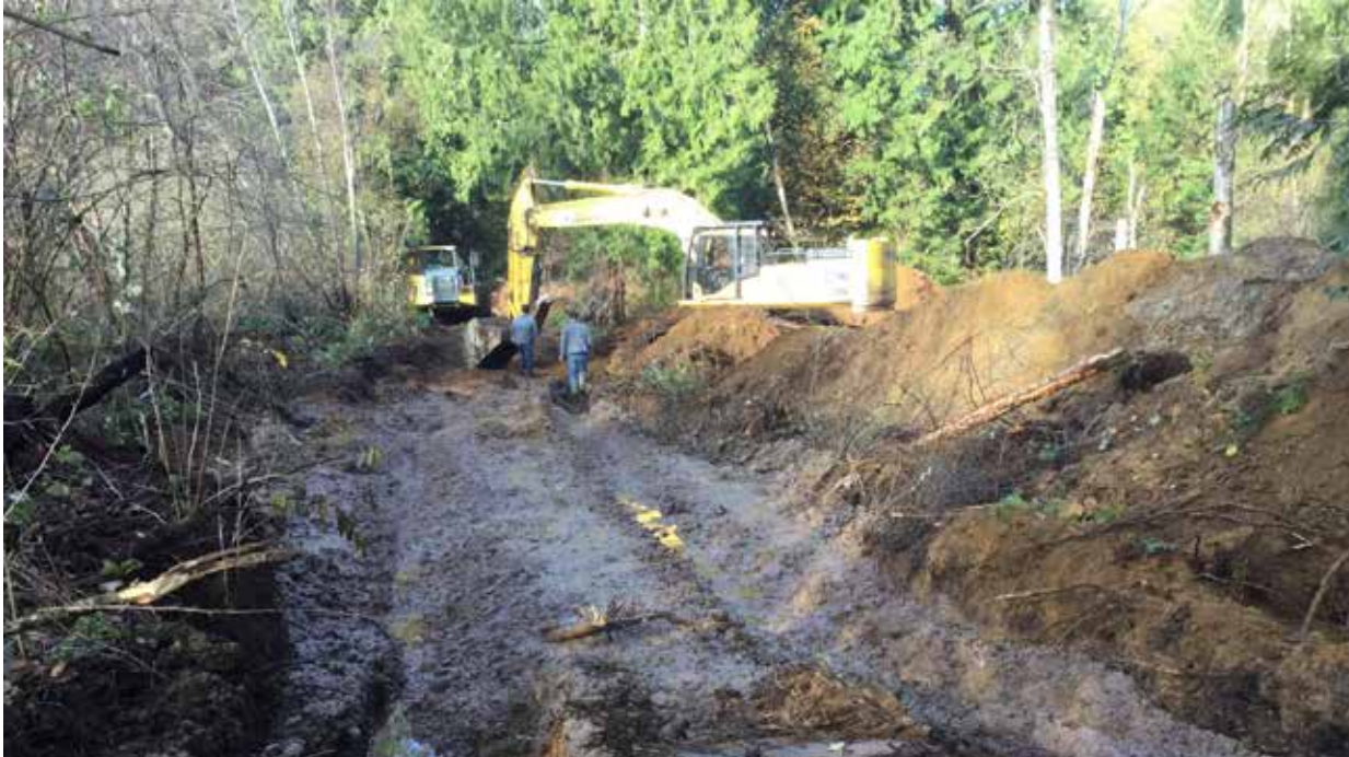
Photo 11 October 28, 2019 - Marhag construction beginning slough excavation at Nancy Phillips Slough.
