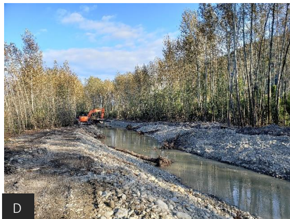
A. Upstream view of groundwater channel being constructed – clearing channel right of way. B. Depth of cut in the dry upstream view. C. Upstream view, groundwater exposed. D. Placing rootwads and LWD to complex the habitat. E. Upstream view after all rootwads placed. F. Retuning chum salmon (bottom left) using the newly constructed spawning habitat.
