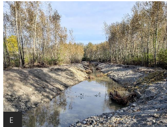
A. Upstream view of groundwater channel being constructed – clearing channel right of way. B. Depth of cut in the dry upstream view. C. Upstream view, groundwater exposed. D. Placing rootwads and LWD to complex the habitat. E. Upstream view after all rootwads placed. F. Retuning chum salmon (bottom left) using the newly constructed spawning habitat.
