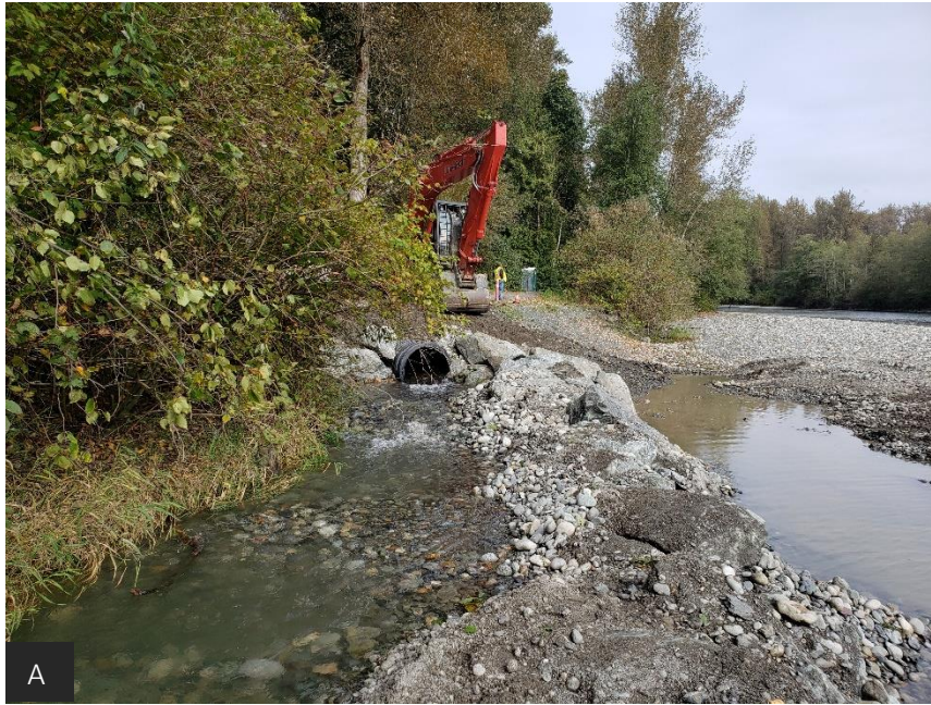
A. 2019 Instream, upstream view of the outlet culvert and stabilized berm. B. Downstream view of the outlet and berm.
