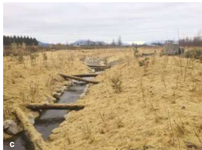
Figure 2. Photo-documentation of instream restoration. A. Installation of the steel connector pipe required to connect McFaden pond to the new Vedder River outlet channel. B. Outlet channel and PVC pipe. C. Straw spread along the project area after construction for erosion and sediment control measures.
