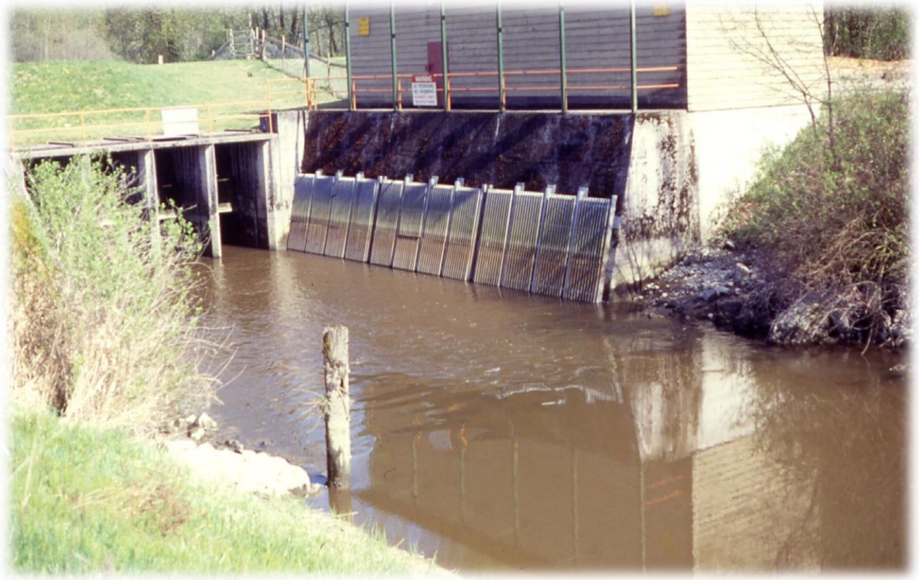
Salmon River Flood Pump Station in Langley, BC, Canada
